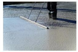
Hoffmann Green have developed the clinker-free cement which involves cold chemical reactions between materials by means of activators, rather than fossil fuel firing used in traditional clinker cement.
